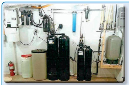
Above is one of the many systems that Garlick's Water Conditioning specializes in. It's a complete system with a CP213 Filter with Oxyblast, a water softener and a Reverse Osmosis system.
